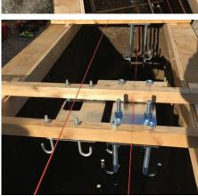
Note: The top of the bolt/tie rod should stick out of the cement at least 2". Keep nut on top of concrete, do not sink in.
