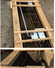
Line up the bolts. Use a string line, template, or other means to ensure bolts are correctly spaced apart. Use the (I) dimension from the project summary. Line up with the other carriage and run parallel to the gate opening.
