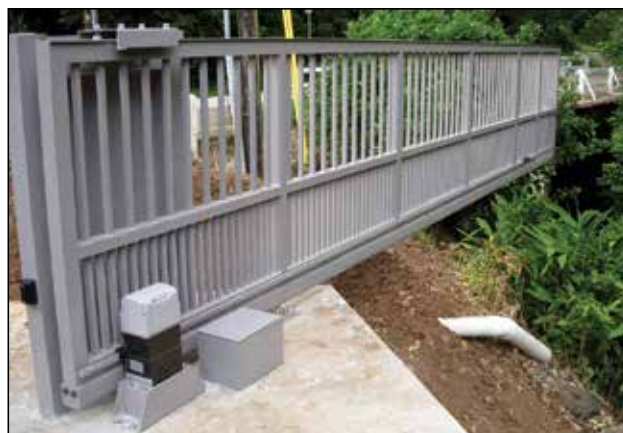
Aluminum sliding gate cantilevering over a slope going down to the river!
